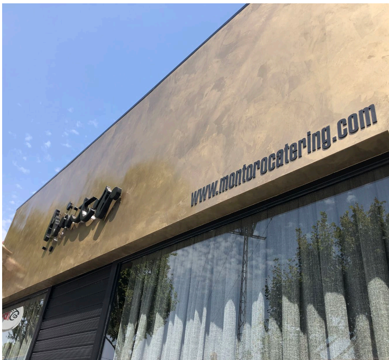
TECNOCEMENTO® METALLIC SYSTEM applied on a restaurant façade in San Juan
